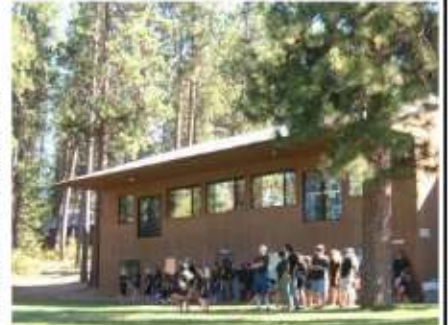
There will finally be a way to get into the dining hall from the backside - and eliminate that nasty drop out the sliding glass doors!
